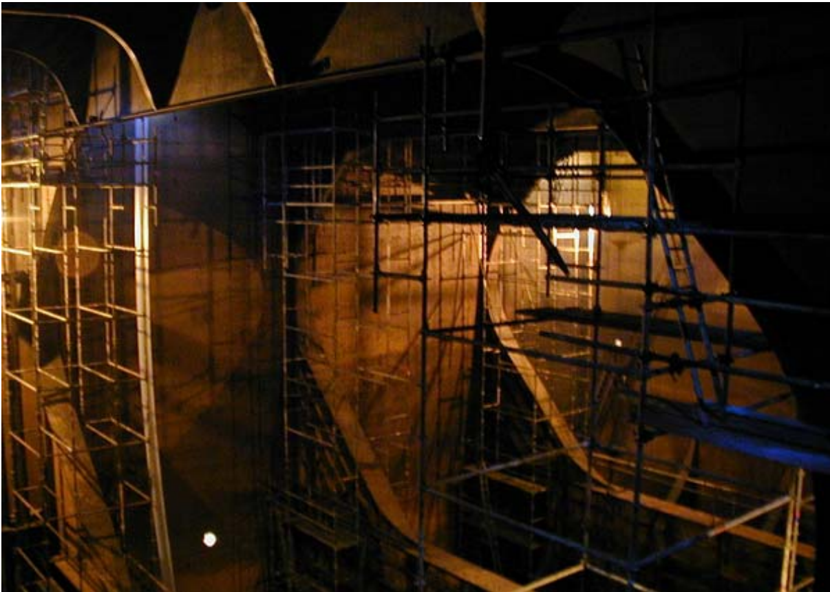
Fig. 4.4.1 Temporary staging during renewal survey of an oil tanker
