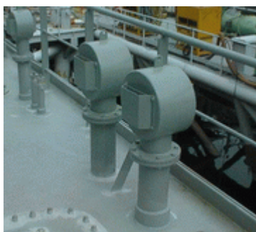
11. All air pipes and ventilators on the fore deck (forward 25% of ship's length), all air pipes to day tanks and selected air pipes and ventilator coamings aft of the forward 25% of the ship's length.
